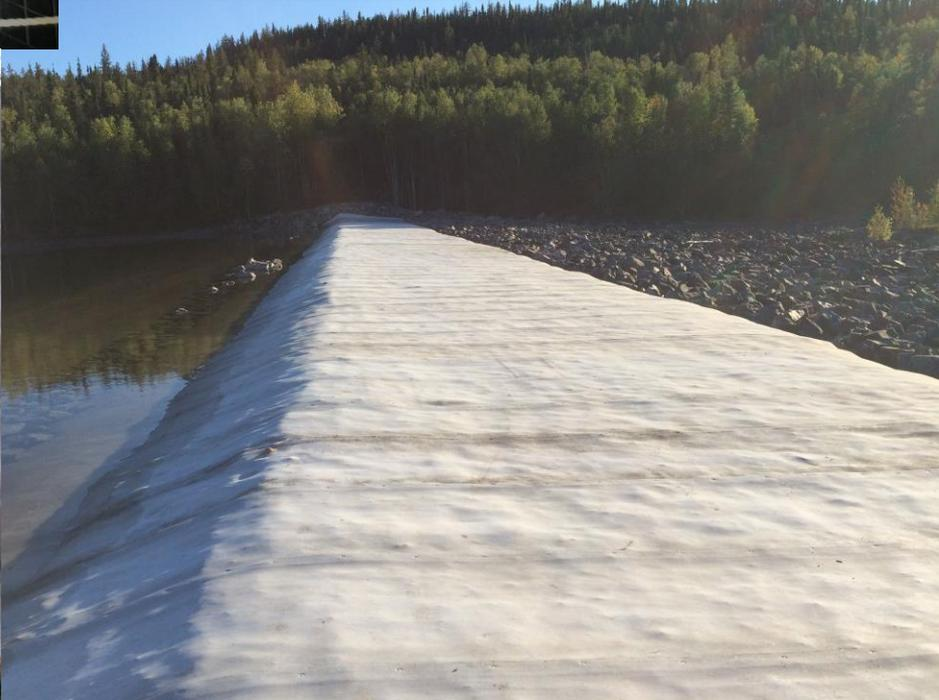
The main spillway is approximately 500m in length with profile sections of 5-8m at 7-15%. The second emergency spillway is approximately 140m in length of varying width at 50% gradient.
